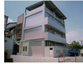
Established GMP standard clean room
